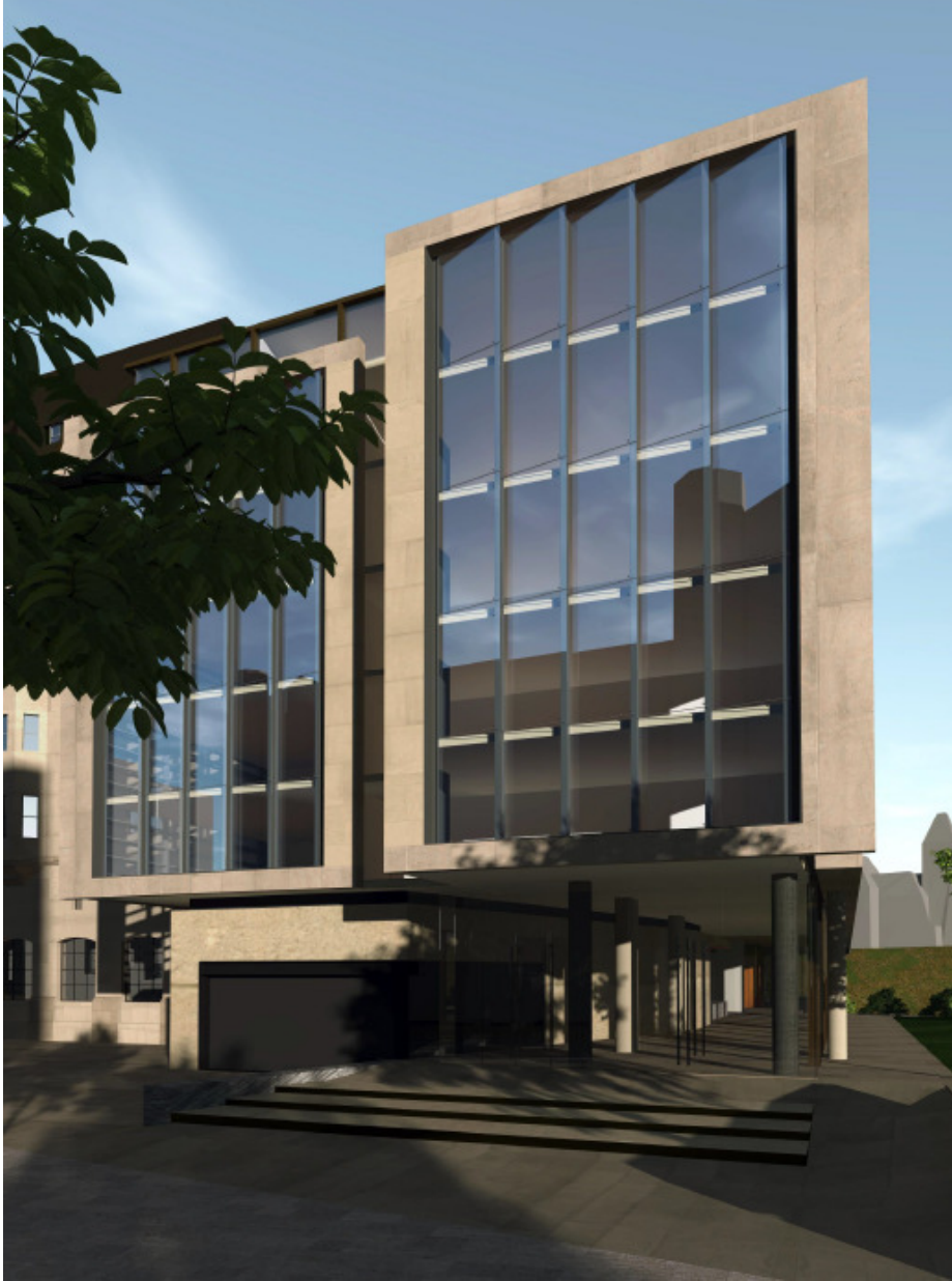
Details, east elevation, showing enclosed gallery, garage doors and glass and bronze panels
