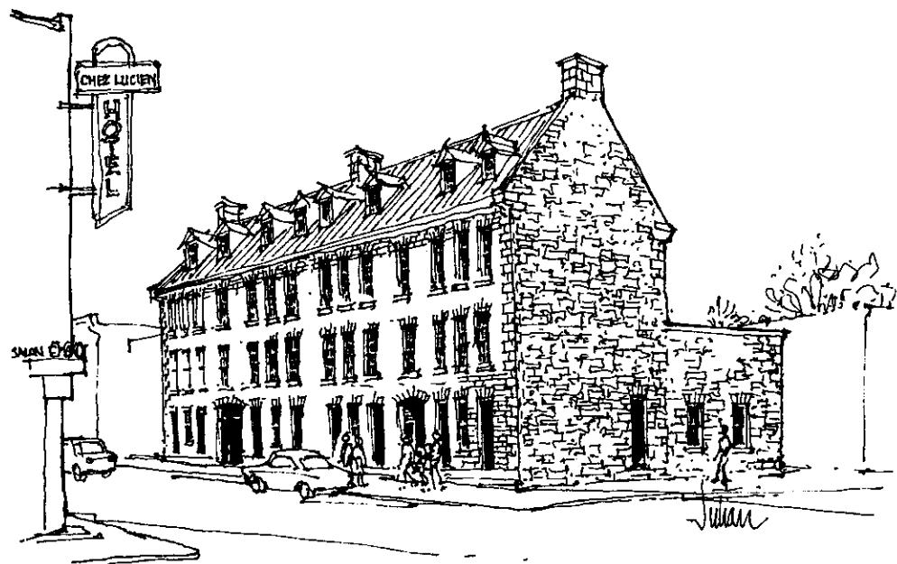
new gable roof with dormers identical to the original will be built. The 28-foot timbers, which were good examples of the capability of Ottawa-Hull's lumber industry in its hey-day, will be replaced by steel beams. On the exterior, two filled-in carriageways will be opened, fire escapes on the façade removed, and double-hung windows installed.
