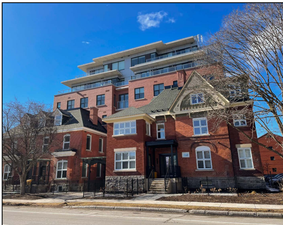
An example of façadism at 282 O'Connor St. Developers preserved the front parts of two Victorian-era houses and built them into a six-story modern mid-rise.
