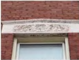
Precast Stone Window Headers to be Restored
