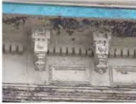
Cornice Dentils & Modillions to be Removed, Restored & Reinstated
