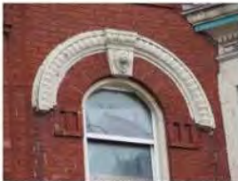
Arched Window Metal Work Details to be Restored
