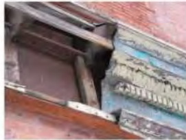
Low Level Cornice to be Replicated
