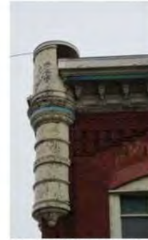
Existing Turret to be Restored, Similar to Original Detailing
